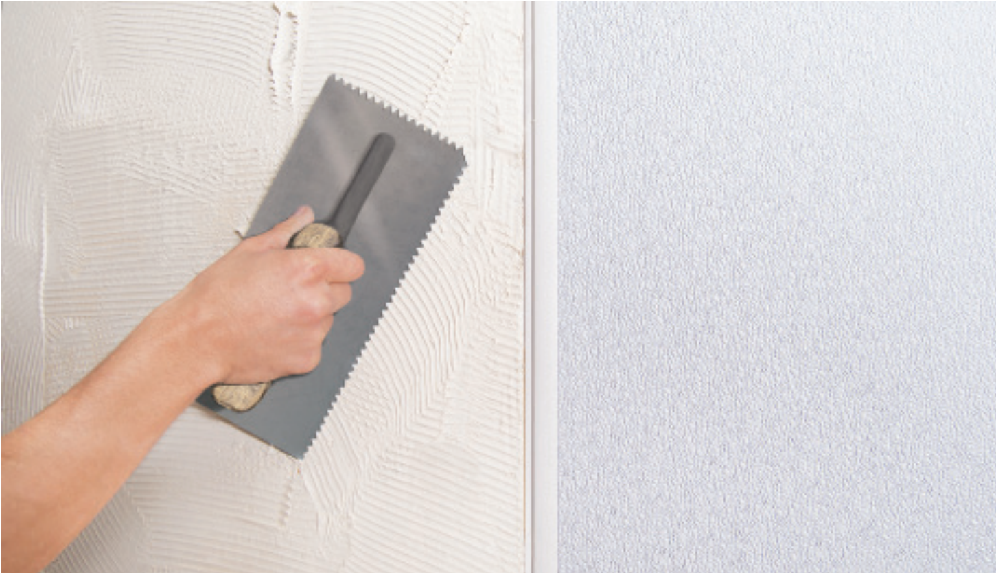
Panel Adhesive Allows new FRP panels to be applied over existing FRP panels
